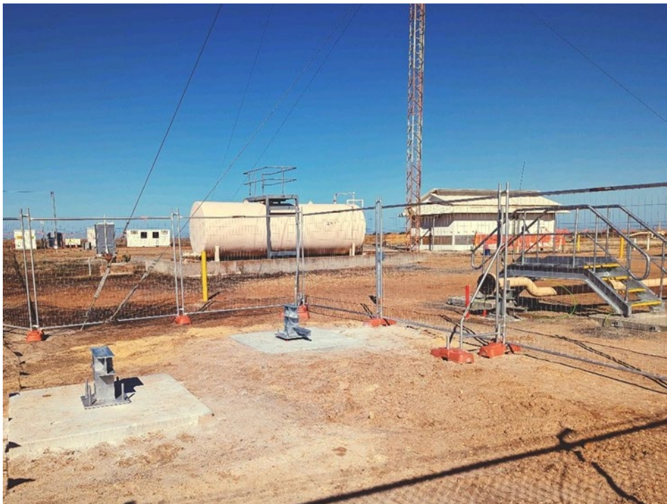
FIGURE 1: PARMELIA GAS PIPELINE TIE-IN POINT
